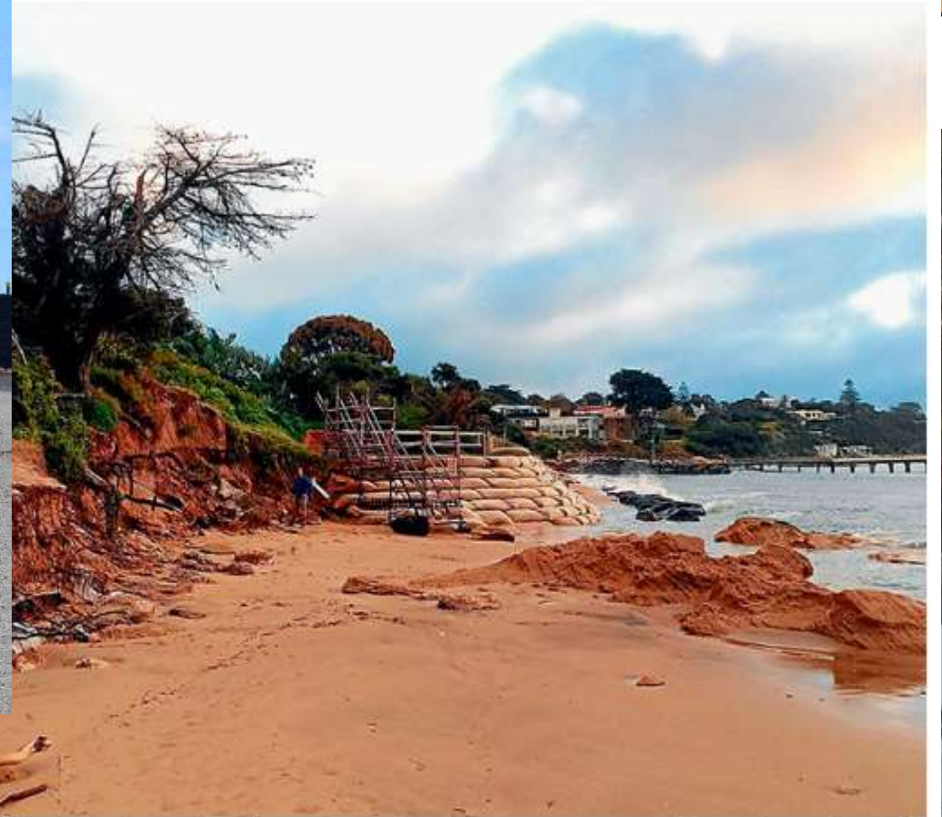
Beach bummer: Windy weather and rough seas last week saw even more erosion of Portsea's once beautiful front beach. Pictures: Josh Clark/Dive Victoria
